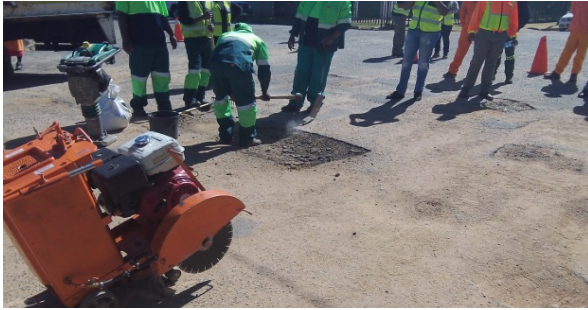
1. CUT / SQUARE POTHOLE WITH PICK
