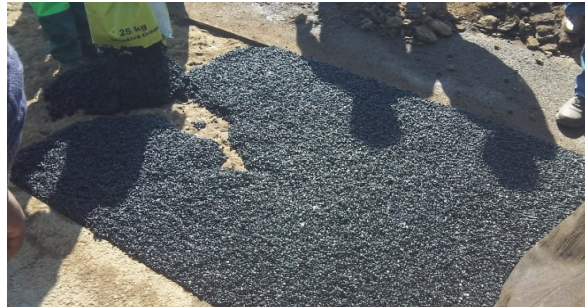
5. FILL HOLE WITH REPAIR COLD ASPHALT
