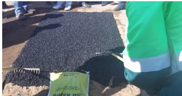
6. RAKE ASPHALT EVEN
