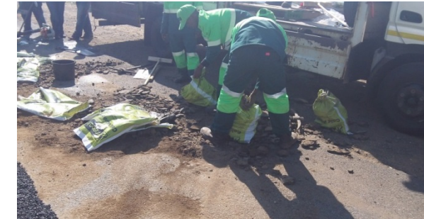
8. FILL EMPTY BAGS WITH DEBRIS
