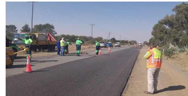
9. OPEN FOR TRAFFIC & MOVE TO NEXT POTHOLE
