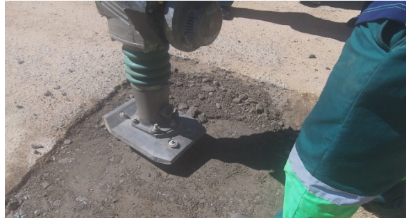
4. COMPACT BASE WITH RAMMER ( Only applicable on deeper holes )
